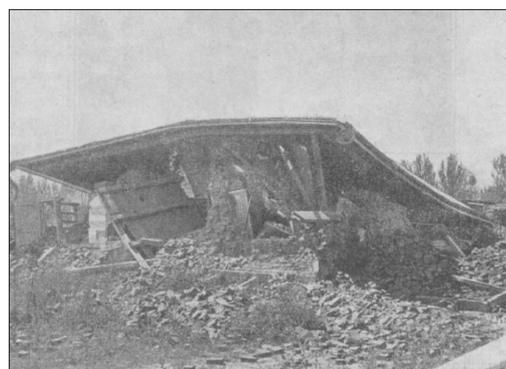
**Fig. 2.** Example of documentation of damage in Verniy (photos from Mushketov, 1890). We can clearly see the type of construction and damage.
