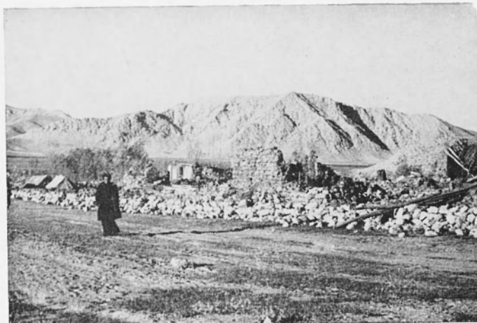
FIG. 5 - Typical adobe-brick houses at Naghan, which completely collapsed.
