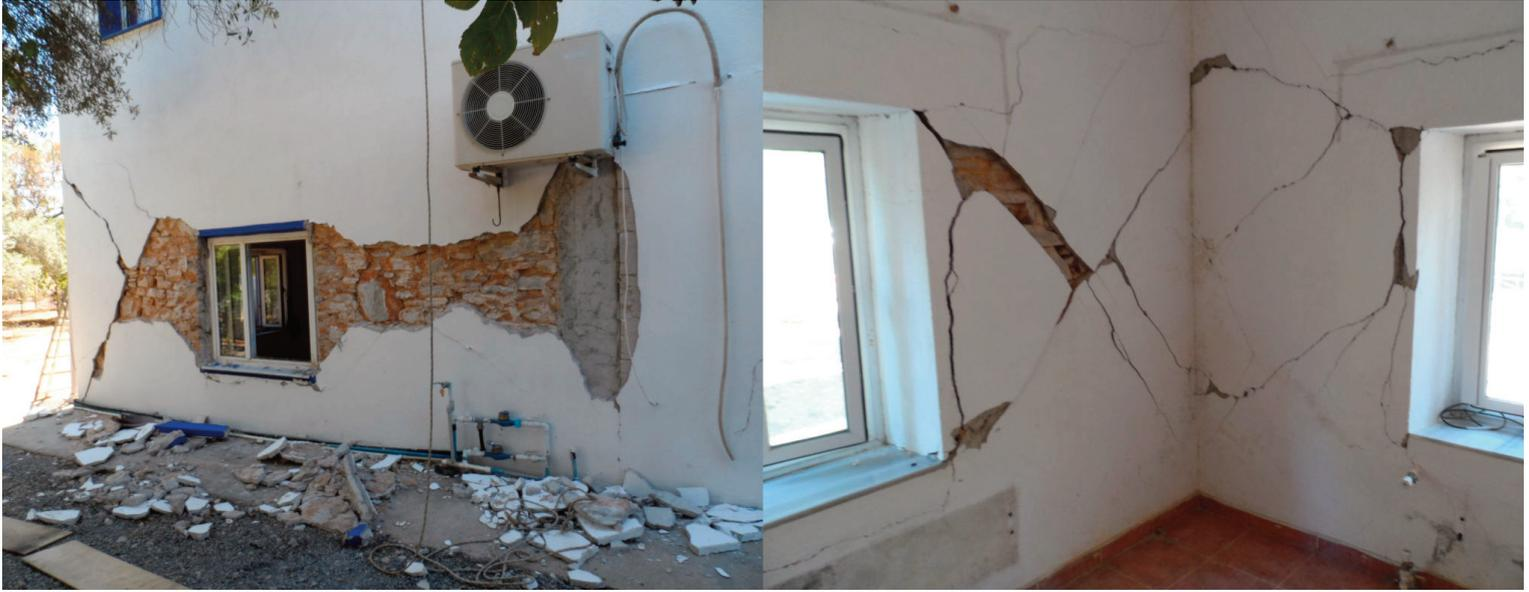
**FIGURE 9.** Heavily damaged 3-storey stone masonry building at the Kizilagac village (Yali). Typical earthquake damage: falling of plaster and shear cracking of the walls.
