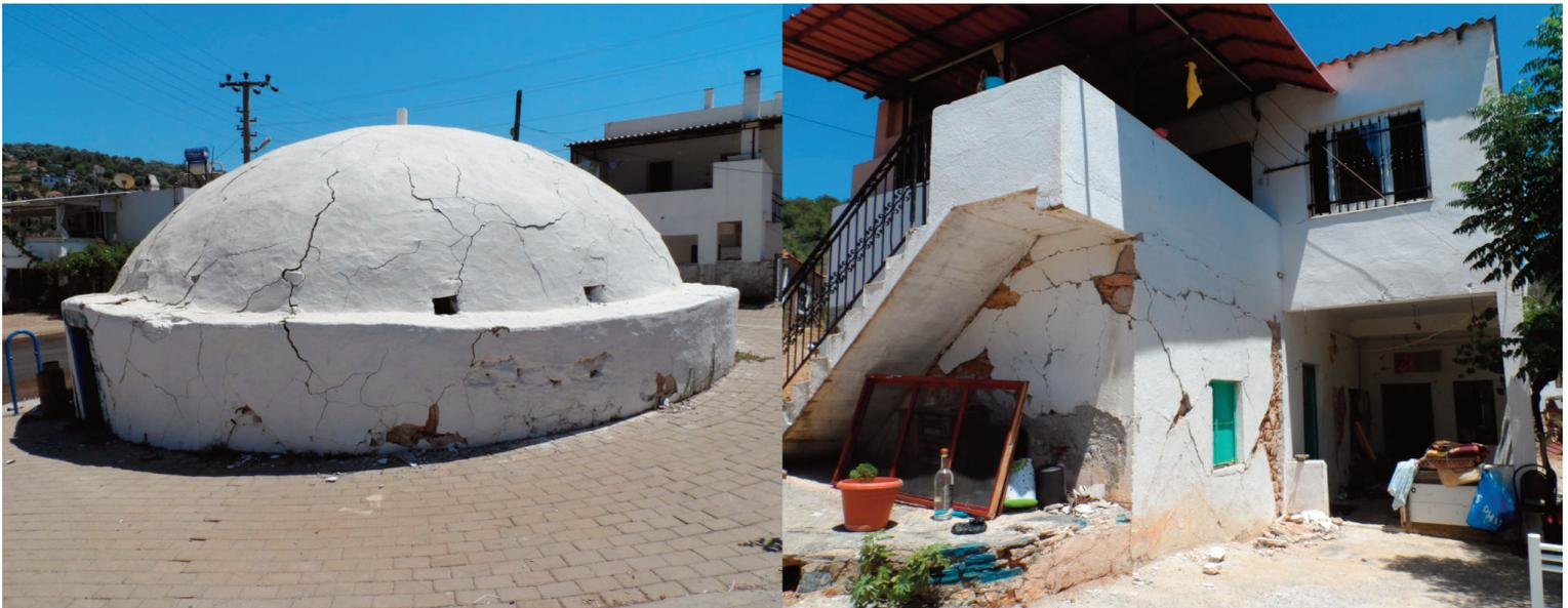
**FIGURE 10.** (left) Damaged traditional dome-shaped water cistern on the road of Ciftlik village to Bodrum centrum; (right) Shear cracking of masonry walls of a house, with upper floor added, at the same village.
