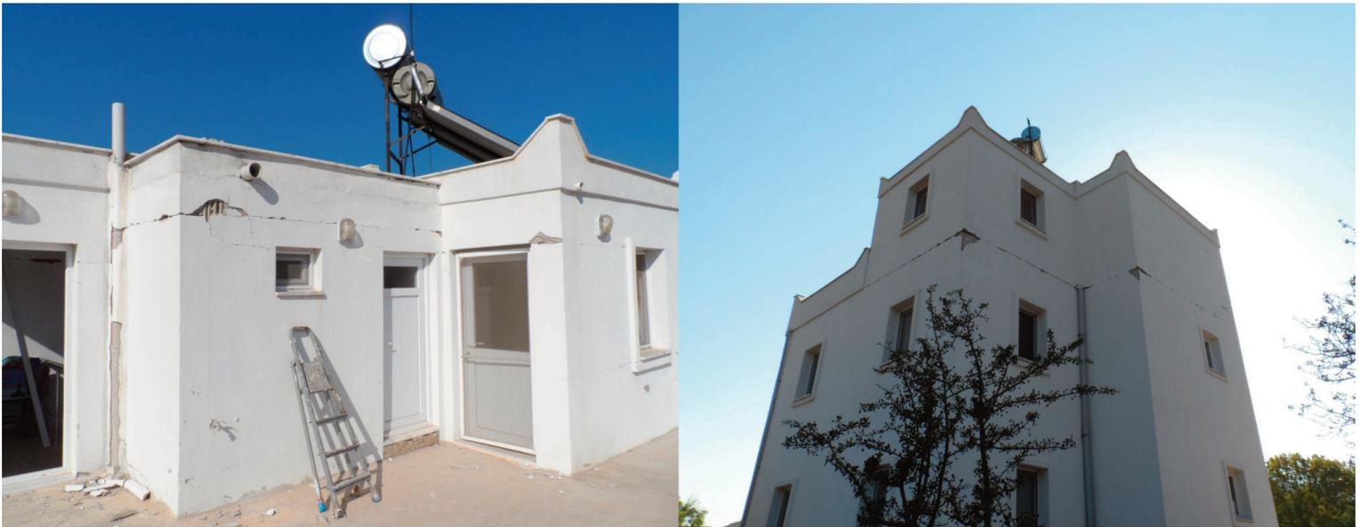
**FIGURE 12.** An unreinforced masonry roof floor built contrary to relevant regulations onto an existing two-storey reinforced concrete building (from an area close to Turgutreis).
