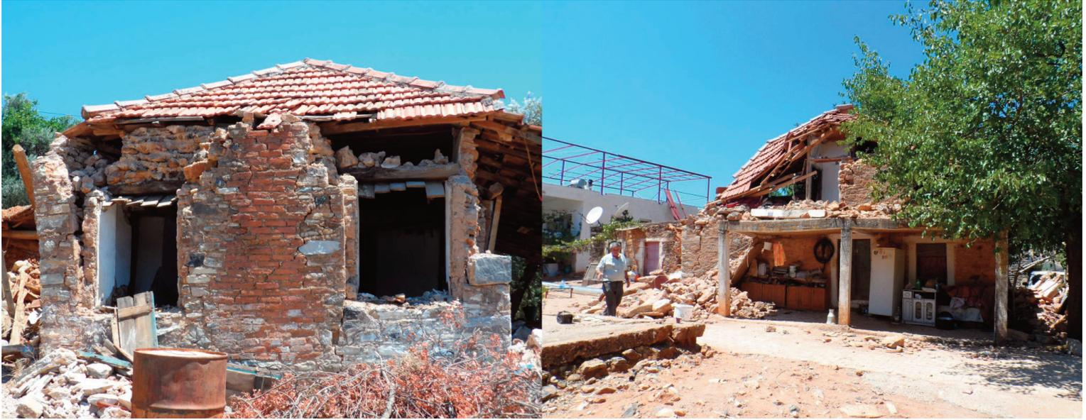
**FIGURE 11.** (left) Partial collapsed of a single-storey stone masonry house in Ciftlik village (Yali). This picture is a good example to common failures of unreinforced masonry systems: diagonal cracking; vertical cracking at the corner joint and out of plane failure; (right) Collapsed houses at the same village.
