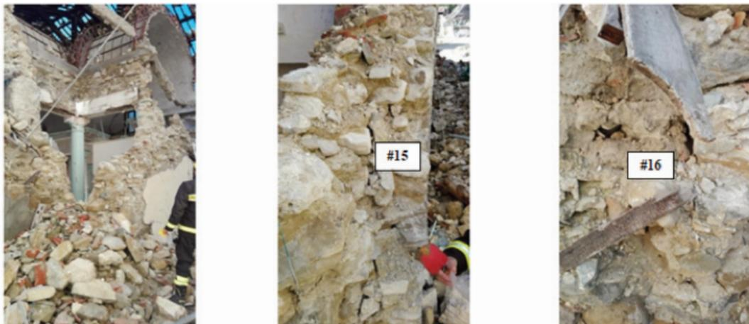
FIGURE 8. Mortar sampling campaign in Pretare – St. Rocco Church (Arquata del Tronto).
