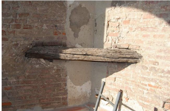
**FIGURE 3.** Wooden chain inserted in an internal corner of the belfry of the Church of San Lorenzo in Borgo San Lorenzo (FI).
