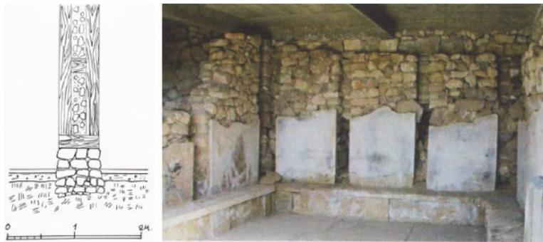
**FIGURE 1.** On the left reconstruction of a wall in Tyllissos with stone socle, timber frame and rubble filled interior [Shaw, 1971]; on the right timber traces in the Hagia Triada villa [Tsakanika and Theohari, 2009].
