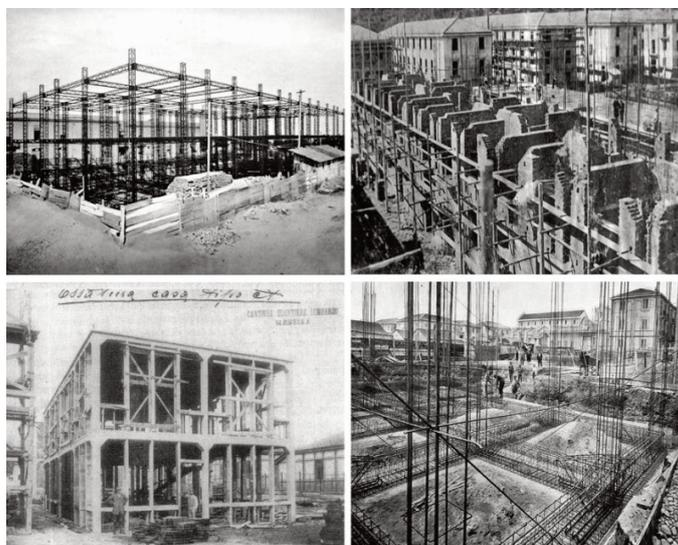
**FIGURE 2.** Construction systems for “anti-seismic” structures permitted after 1908 Messina earthquake: frames of steel (1909 et seq.); reinforced masonry (from 1912 to 1924); reinforced concrete frames with diagonal bracings (1909); frames in reinforced concrete with rigid knots (1909 and then since 1924).
