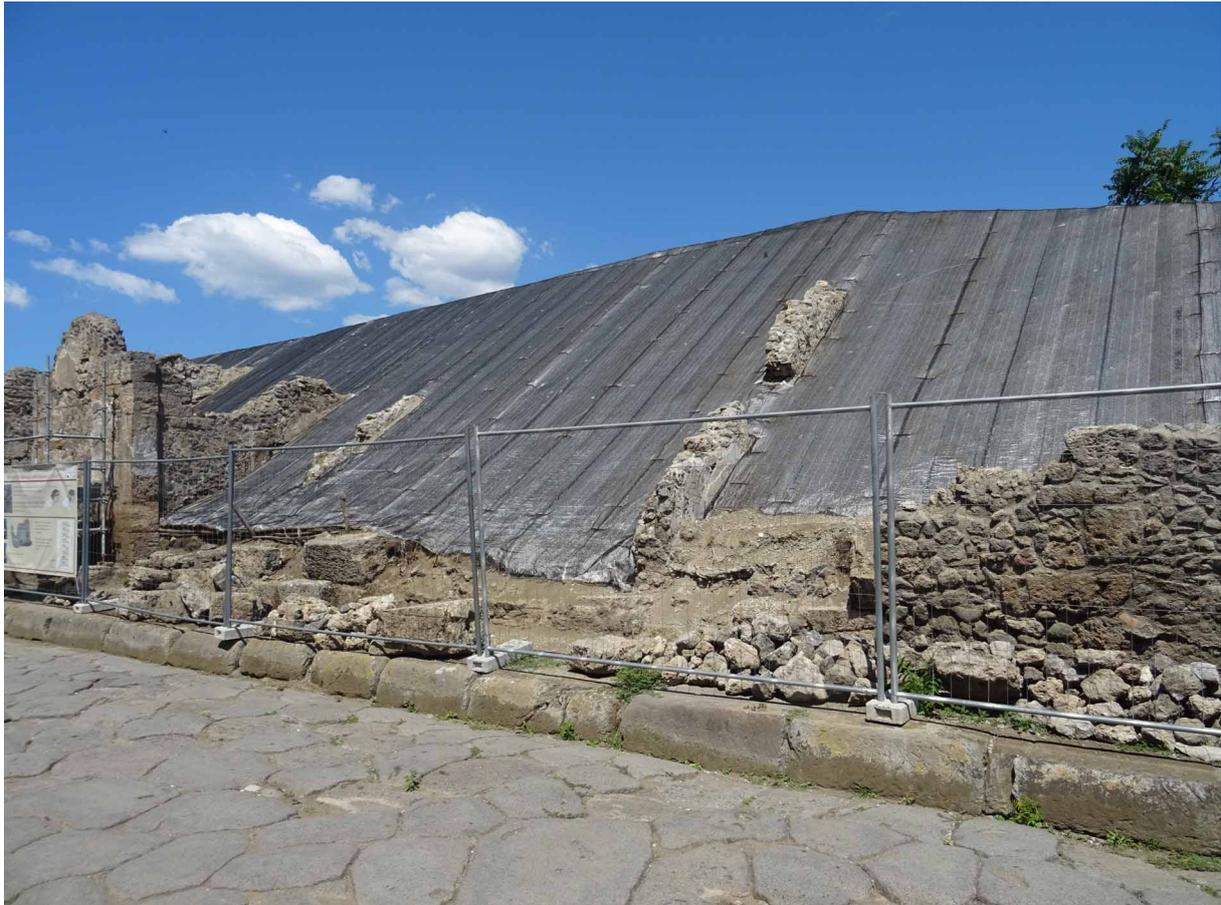
**Figure 3.** The volcanic products around the excavation were covered with geomats during the recent works to make safe the perimeter of the site.
