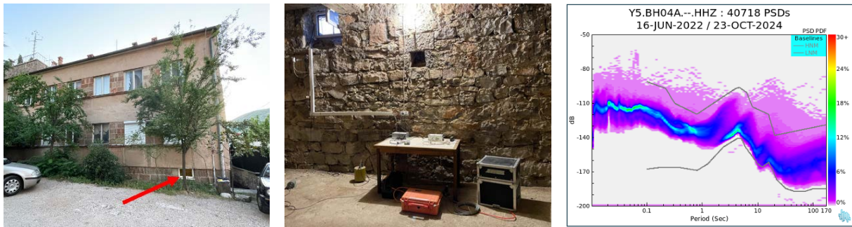
Figure A4. BH04A, Mostar, is installed in the Meteorological Observatory Mostar. The sensor is located in the basement, in the northeast corner of a two-storey office building. The basement is unused. The sensor is placed directly on the concrete floor of the building in a dense urban area.
