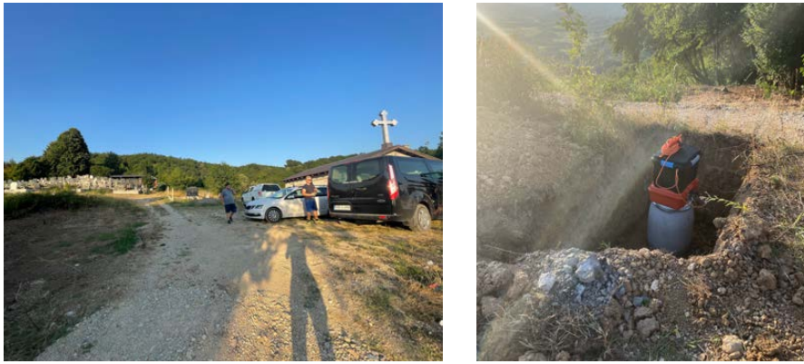
Figure A19. BH19A, Zvornik, is installed in an open free-field. The sensor is inside a self-constructed seismic vault on a concrete foundation. The ground consists of soil. Mobile phone coverage is very limited despite a nearby cell tower, resulting in the recovery of minimal data.
