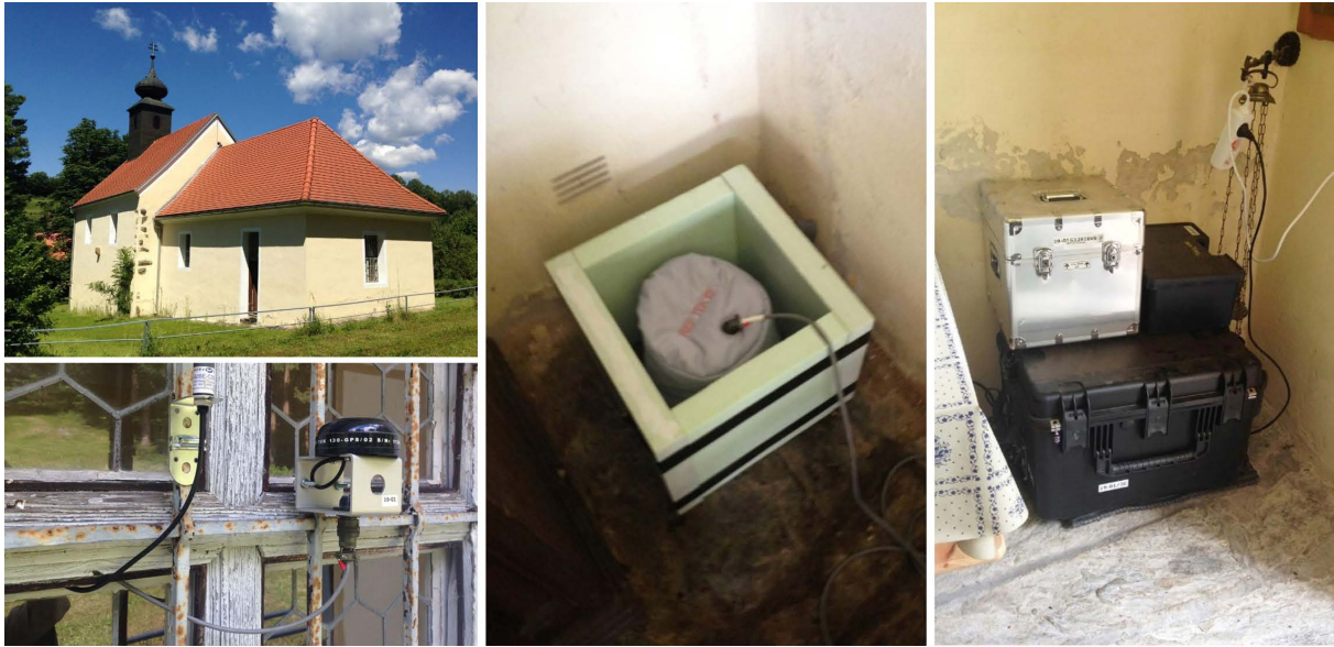
Figure 6. Example of the installation of temporary stations in Austria: outside and inside views of station A011B Reinberg.
