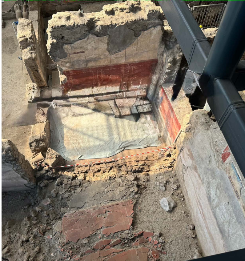
Figure 7. Wall collapsed onto the floor (below) in the House of the Second Colonnaded Cenacle. The red plaster and light-colored baseboard, like those still upright, correspond to the interior face of the wall.
