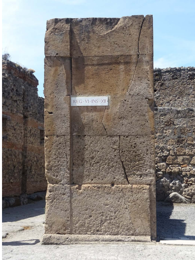
Figure 11. Tuff blocks with visible fractures in the wall of the shop (VI,12,1), connected to the House of the Faun.
