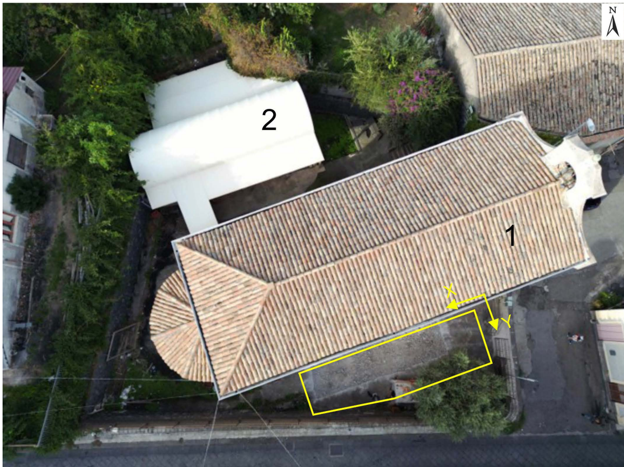
Figure 3. Location of the GPR survey conducted within the church courtyard (area marked by the yellow box). 1) Medieval church of Maria Santissima Annunziata; 2) Paleo-Christian basilica.
